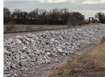
Completed section in IA
