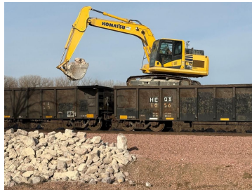
Placing rip rap in SD
